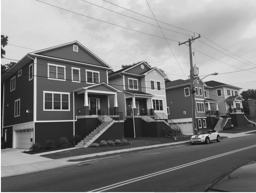
FIGURE 9.4 New construction on the east side of the 200 block of Charles Street in the Darbytown neighbourhood © Christine R. Henry and Andréa L. Smith, August 2018
